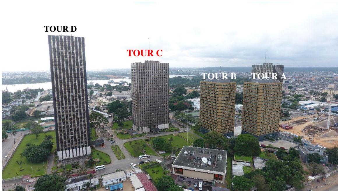
Figure 28: Infrastructures proches de la TOUR C
